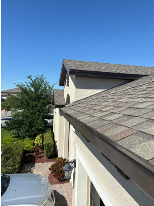
Roof Covering Material Asphalt composition shingles.
