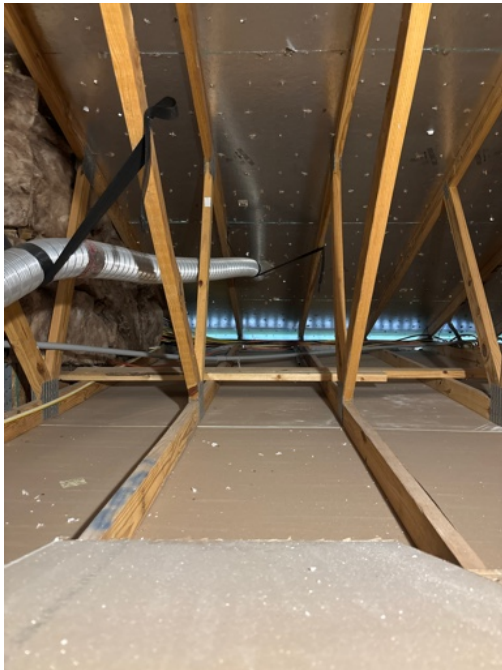
Attic Ventilation Type Ridge Vents and soffit vents
