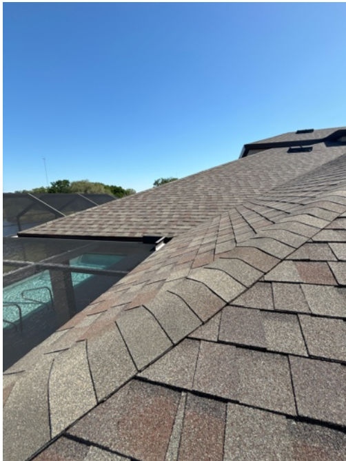
Roof Covering Material Asphalt composition shingles.
